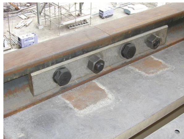
Photo 2. Fe-Mn-Si SMA fish plates for crane rails
